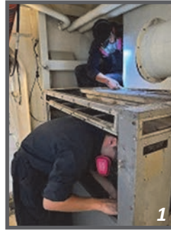
Left: STG2(SW) Johnny Cabrera (top) works on removing one side of the supply air ducting from the fan coil assembly while STG2(SW) Daniel German (bottom) starts unbolting the upper from the lower cabinet.
