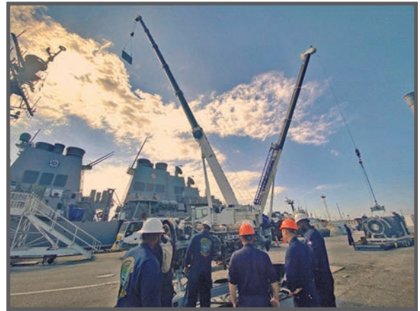
Both cranes hard at work! Left reinstalling silencer's on 1A, and right preparing the old 2A GTM for transport.
