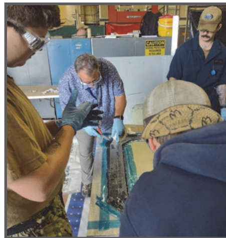
CNRM Team Lead Timothy Jones (center) demonstrating the proper method of applying the Stop-Sign Edge Sealer cloth to the MARMC Team members. (Photo by Andy “Rusty” Vasquez.)
