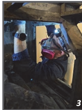
STG2(SW) John Lukashonak removes the final fasteners of the supply air ducting from the air outlet port on the fan coil assembly.
