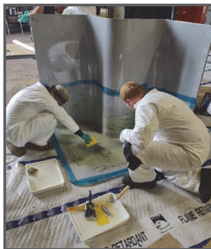
MARMC team member Caleb Grimes and Gougeon Brothers Advisor Don Gutzmer installing the 5th layer of Fiberglass on an outward corner of the mockup patch. (Photo by Andy “Rusty” Vasquez.)
