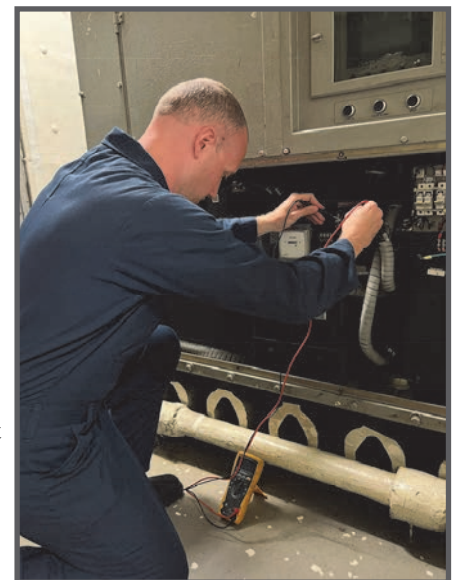
EM2 Richard Cooper troubleshooting one of the Aircraft Electrical Servicing System Frequency Converters. (Photo by Kat Ciesielski.)
