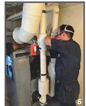
STG2(SW) Daniel German cleans and prepares a return duct for future installation.
