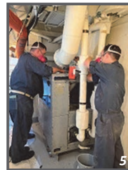
STGC(SW/IUSS) Mark D. Moles (left) works on removing vent duct bolts while STG2(SW) Daniel German (right) prepares a return duct for future installation.
