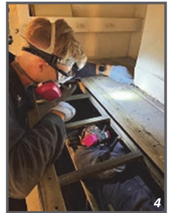
A few fasteners required two people to remove. STG2(SW) Johnny Cabrera (right) holds the riveted nut in place while STG2(SW) John Lukashonak (left) turns the bolt.
